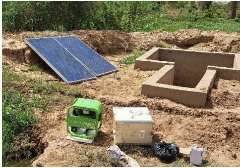
The basin, two of the four solar panels and the aQysta solar pump on HortiHub Land.
